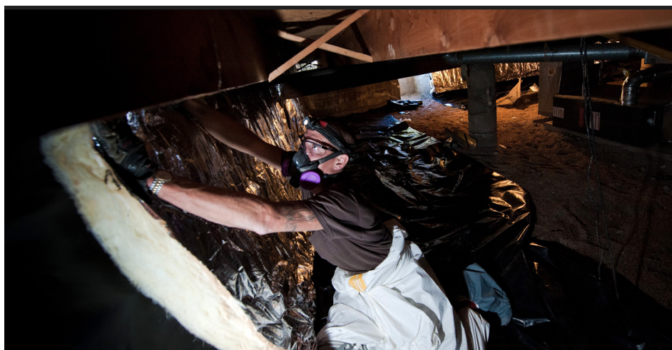
Installation of moisture barrier and insulation as part of the Federal Weatherization Assistance Program. Photo courtesy of the US Department of Energy
